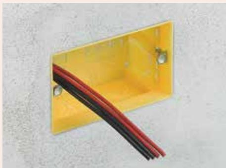
Do not leave the wired devices hanging out of the boxes, during building yard work
